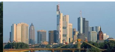
German Office Frankfurt/Main GERMANY
