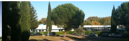
POWERSYS Corporate headquarters Le Puy-Sainte-Reparate (Aix-en-Provence) FRANCE
