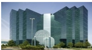
POWERSYS Inc Southfield, MI
